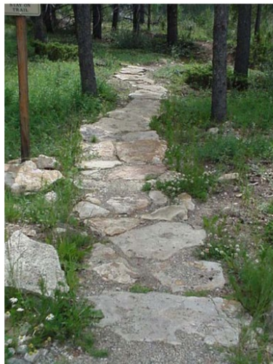
Armoring on the Lower Flume Trail.
