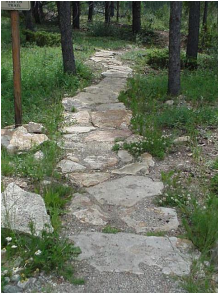
Armoring on the Lower Flume Trail.
