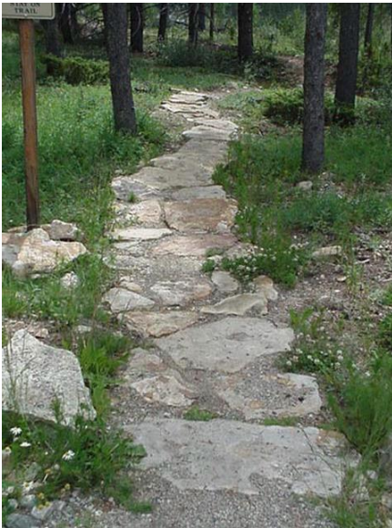
Armoring on the Lower Flume Trail.
