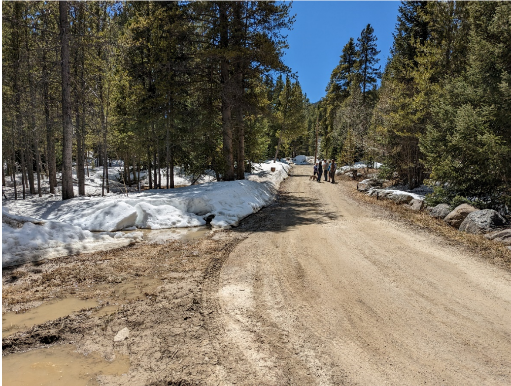
Figure 9. Looking west along Blue Grouse Trail. Nuisance flow ponding at lot 101/102 was observed.
