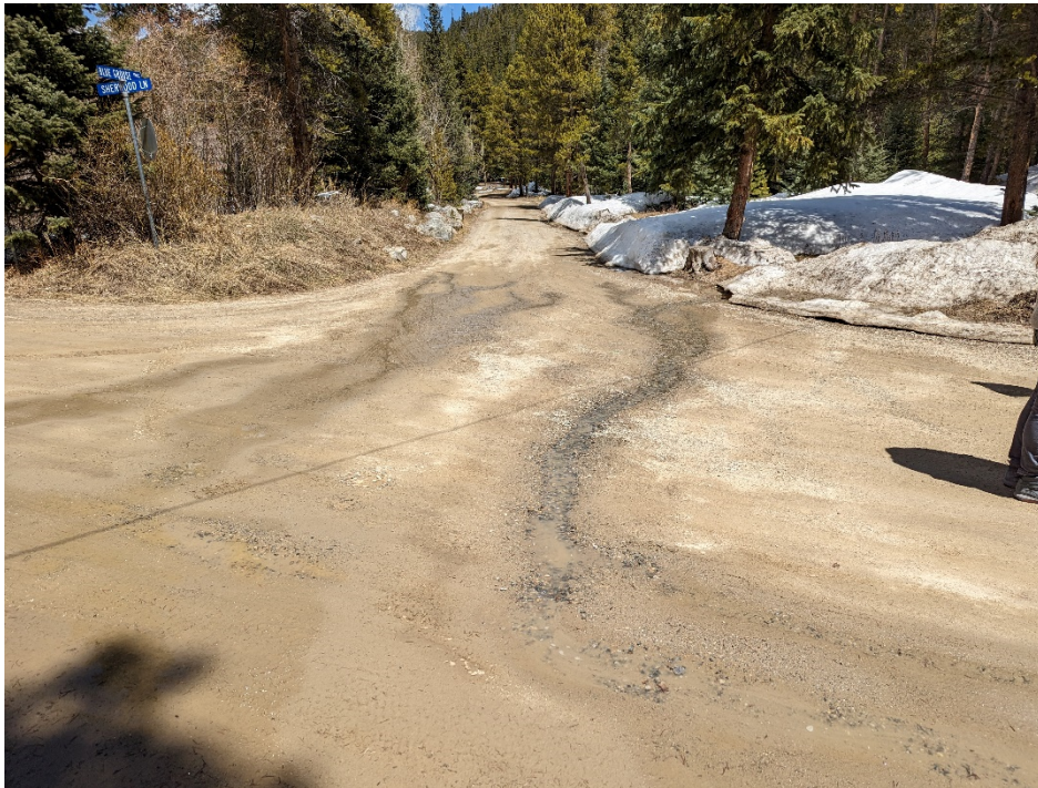
Figure 8. Intersection of Sherwood Lane and Blue Grouse Trail. Looking east down Blue Grouse Trail. Nuisance flows overtopping Sherwood Lane and continuing along Blue Grouse Trail were observed.
