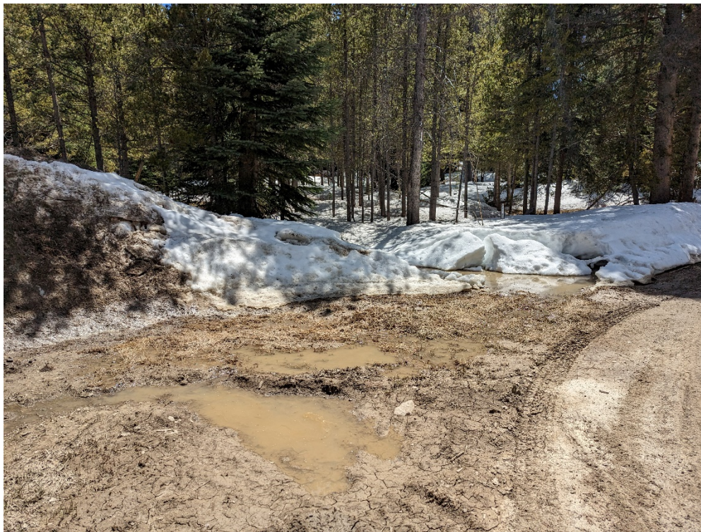
Figure 10. Ponding from nuisance flows at lot 101/102 was observed .
