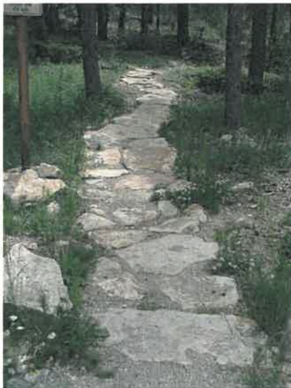
Armoring on the Lower Flume Trail.
