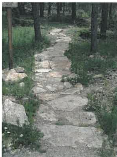
Armoring on the Lower Flume Trail.
